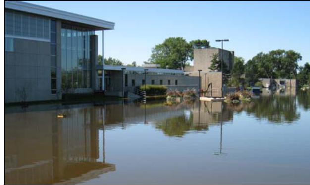
Figure 1. Flooding of the main parking lot on the north side of campus. (Photo by E.P. Argyilan)
